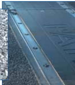
Bending Plate Installation
