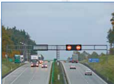
Traffic Management on A4 Motorway Poland
